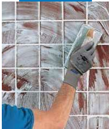
Laying the product with a rubber float
