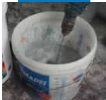
Slowly add component A (powder) while stirring with a mechanical mixer, keep stirring slowly until a perfectly homogenous mix is obtained
