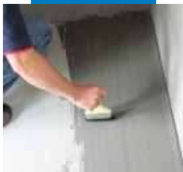
Applying K11 High Flexible Waterproofing Slurry
