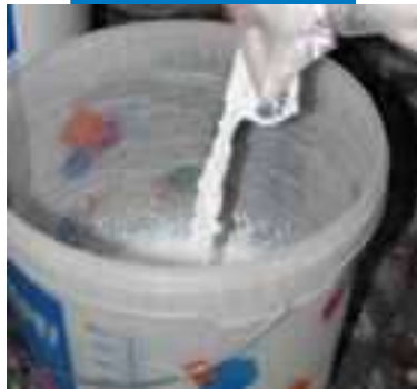
Pour component B of the appropriate amount into a mixing container
